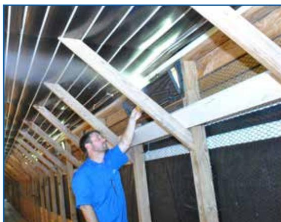
When smoke testing a house, it is advisable to do it under “worst case” conditions. That is, when the house is at brooding temperature and the ambient temperature is at, or close to, as cold as it may get.
