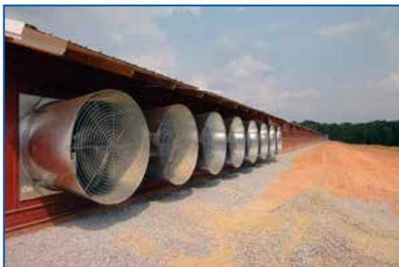
The air inlets should be situated at the opposite end of the house from the tunnel fans. These should be of equal size (area) in each sidewall of the house. The tunnel ventilation inlets are usually closed using some sort of hinged door or curtain system. Closing of the inlets must be automated and linked to the control system.
